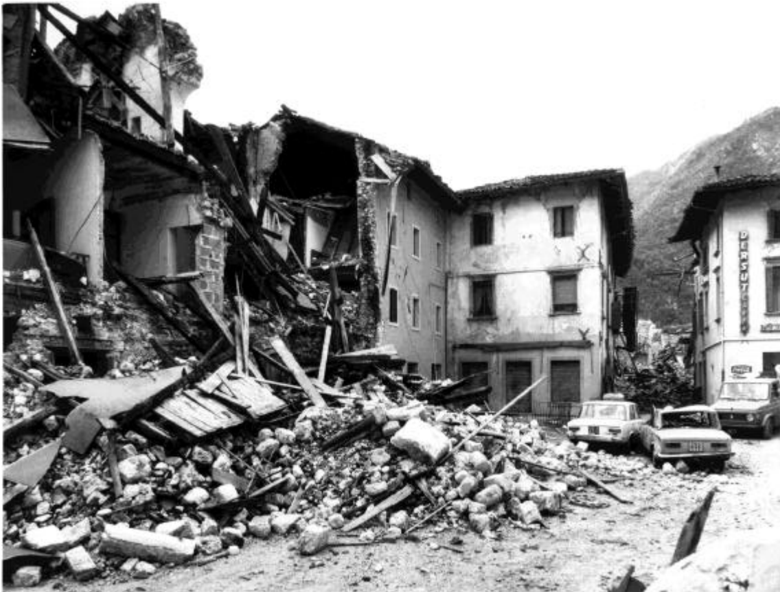
Figure 5b: Venzone town - Building n. 47.
