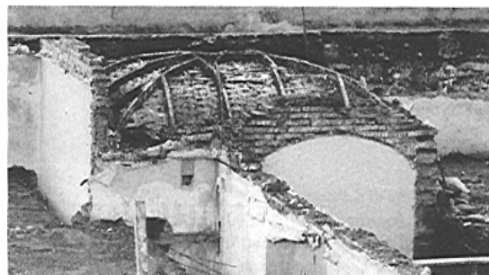
Figure 9.9 - Upper surface of a “false” vault (Randazzo, 1988).
